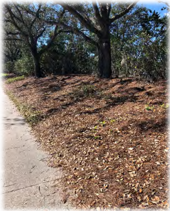
Missing SOD Strip at Side Walk
